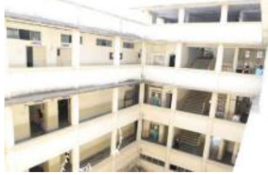
F- WING STAIRCASE AND CIRCULATION AREA
